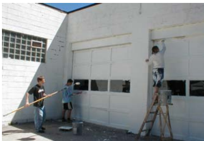
Charlevoix teens give the building a fresh coat of paint.
