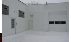
Garage - elimination of one garage door, install entry door, furnace room, new boiler for hot water heating system, and removal of lots of STUFF!!
