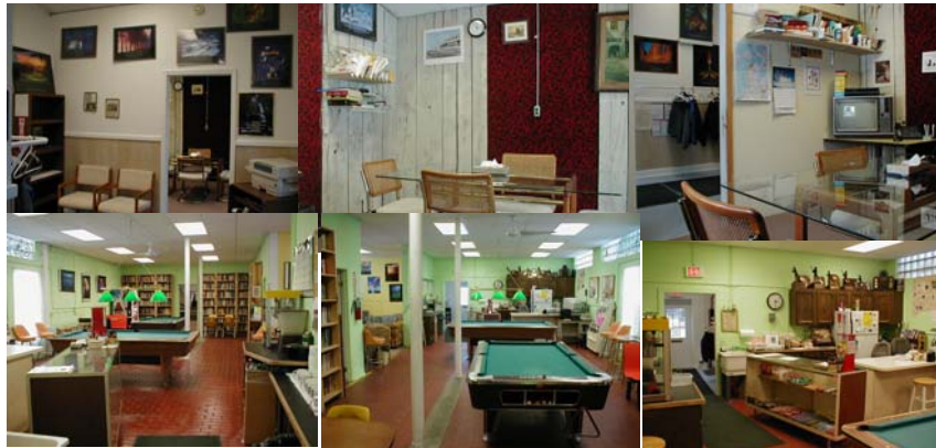
Main Room - installation of sink, cupboards & countertops, replaced old door with window in east wall, drop-in ceilings, ceiling fans, relocated pop machine, painted the walls, removed 4x4 beam to couch room.
